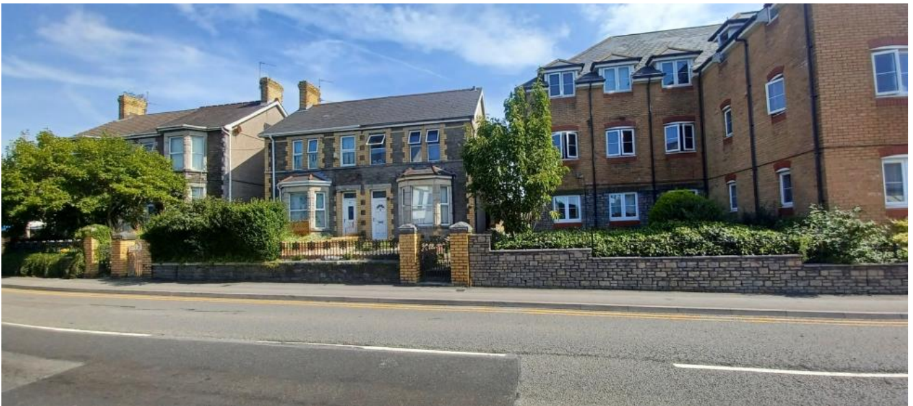
Figure 4 Photographs of the application site Street Elevation View
